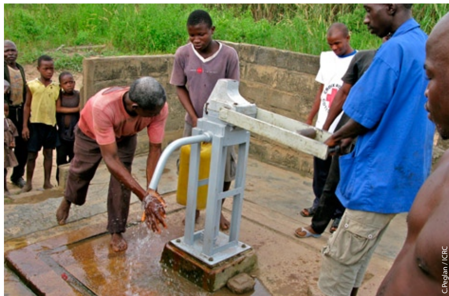
A water hole being repaired at Duékoué
